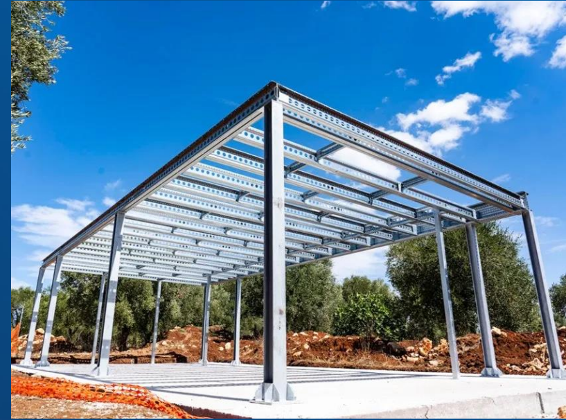
Fig. 4: Steel framed building
