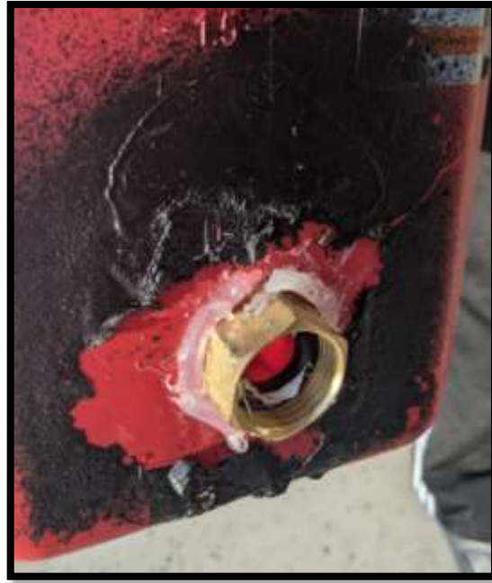
Figure 6: Reservoir pump fitting
