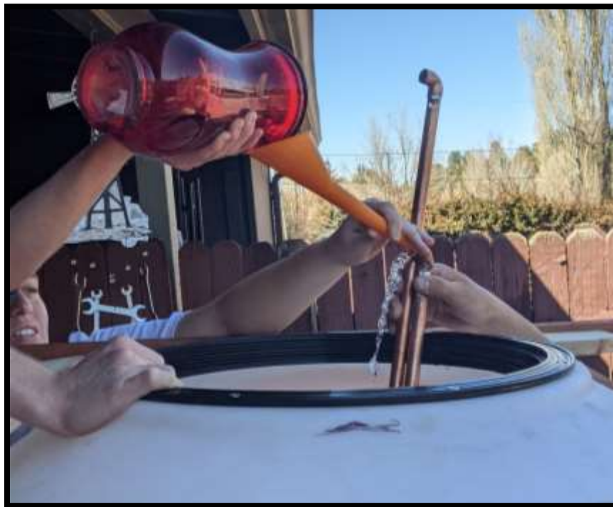
Figure 17: Filling the liquid-to-liquid heat exchanger.
