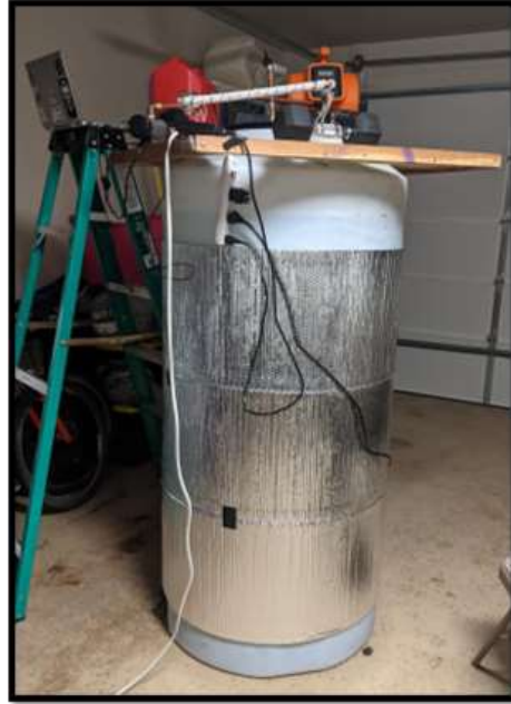
Figure 20: Insulation wrapped around the tank
