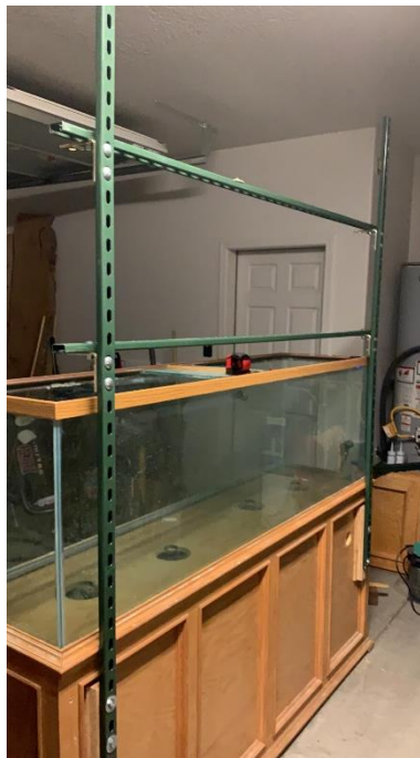
Figure 3: Rear mounted Unistrut
