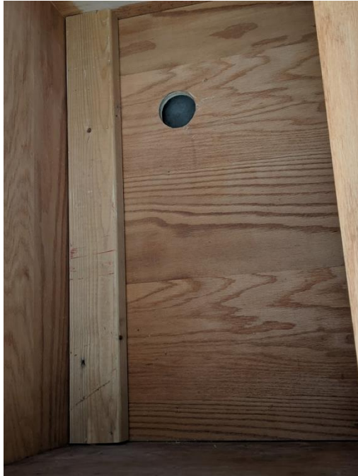
Figure 1: 2x4 Internal reinforcement
