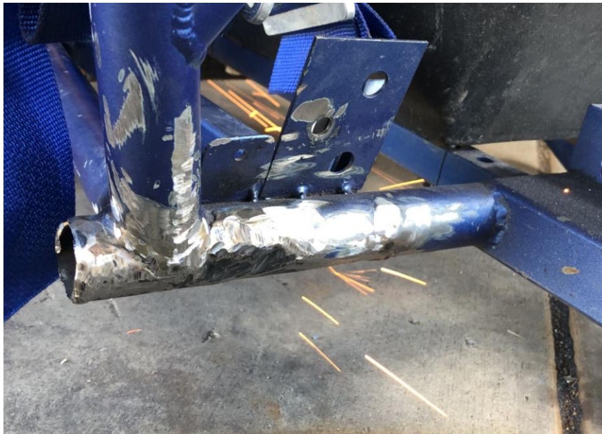
Figure 7. Grinding off trailing arm mount
