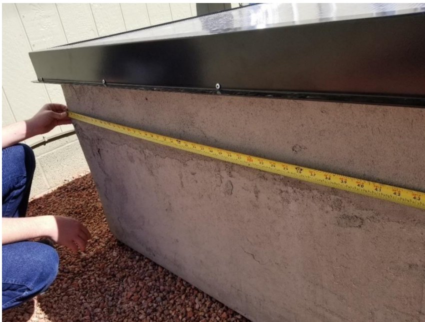
Figure 2: Width Measurement of the Box
