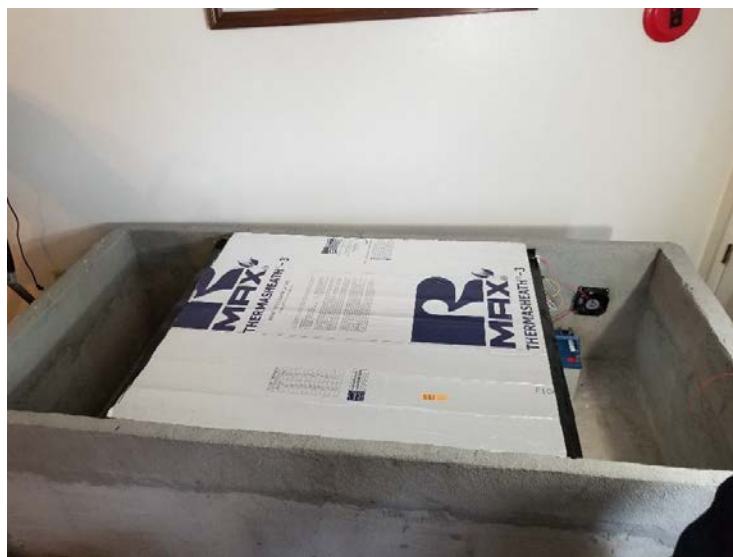
Figure 21: Picture of Thermal box inside Green Rhino Box
