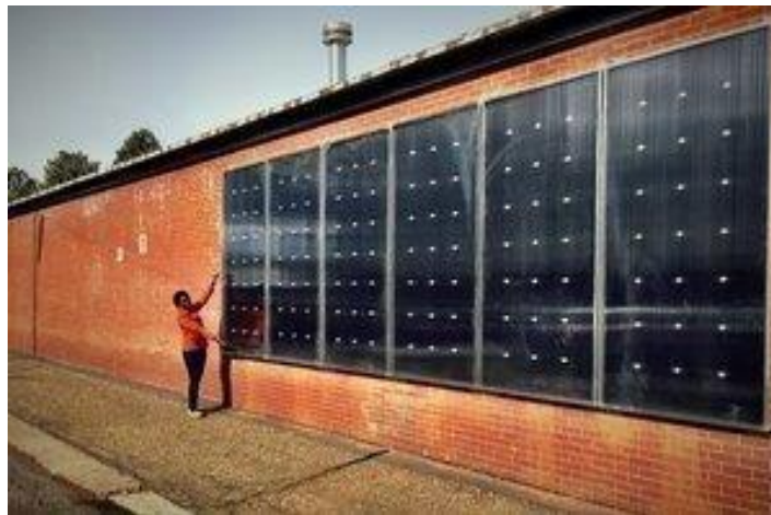
Figure 9: SolarThermiX Solar Air Heater on ROTC Building [2]
