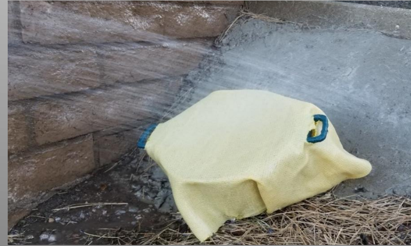
Figure 19. Permeability testing on a test section of HDPE fabric
