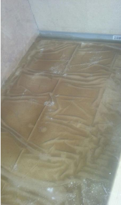
Figure 34: Wrinkles of fiberglass resin
