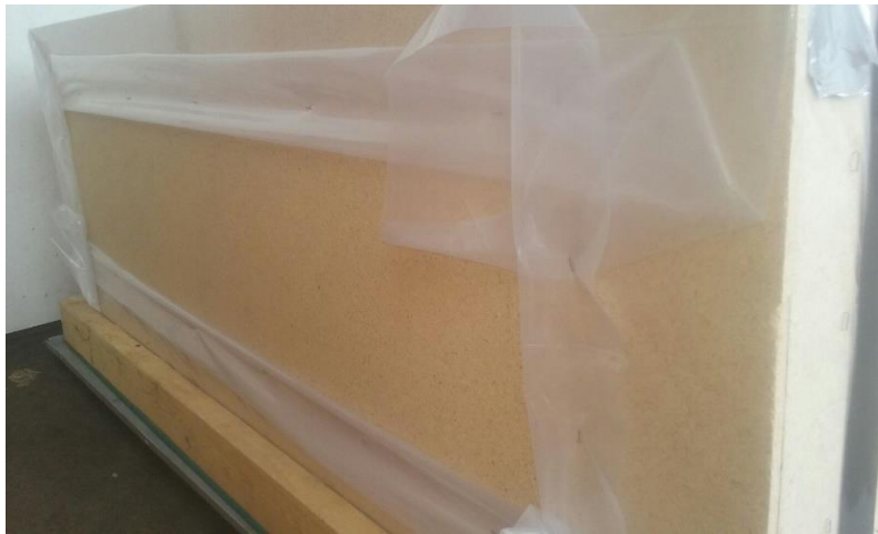
Figure 30: Plastic sheets coverage
