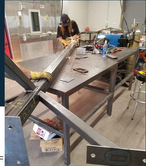
Figure 9: Truss Column Grind
