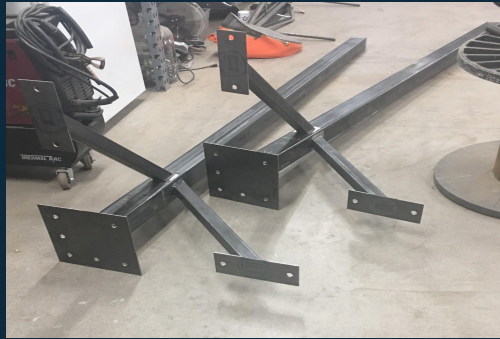
Figure 18: Truss Welded Plates
