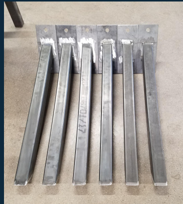
Figure 16: Tacked Steel Truss
