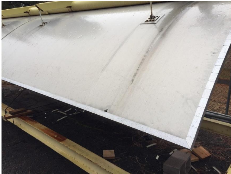
Figure 8 - Installed trim on flat and curved edges
