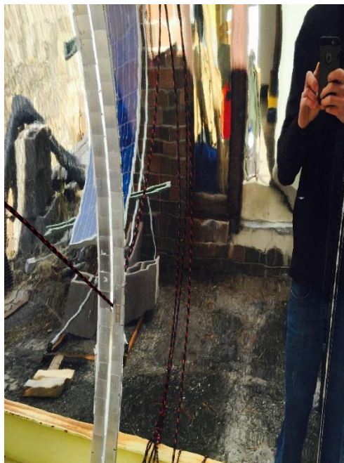
Figure 9- Inner trim installed
