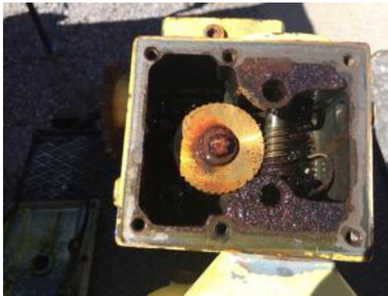
Figure 4: Upper gearbox with the cover off
