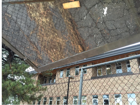
Picture3: Installed Trim
