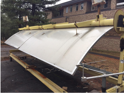
Picture1: Installed Trim
