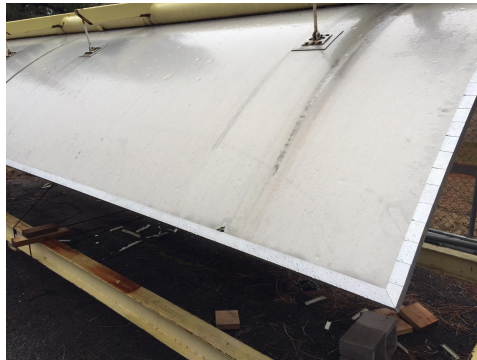
Picture4: Installed Trim
