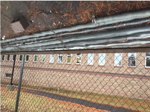
Picture2: Installed Trim
