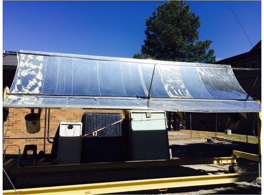
Front View of Energy System
