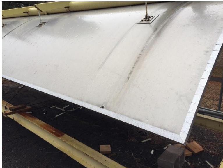
Figure 18 - Installed trim on flat and curved edges
