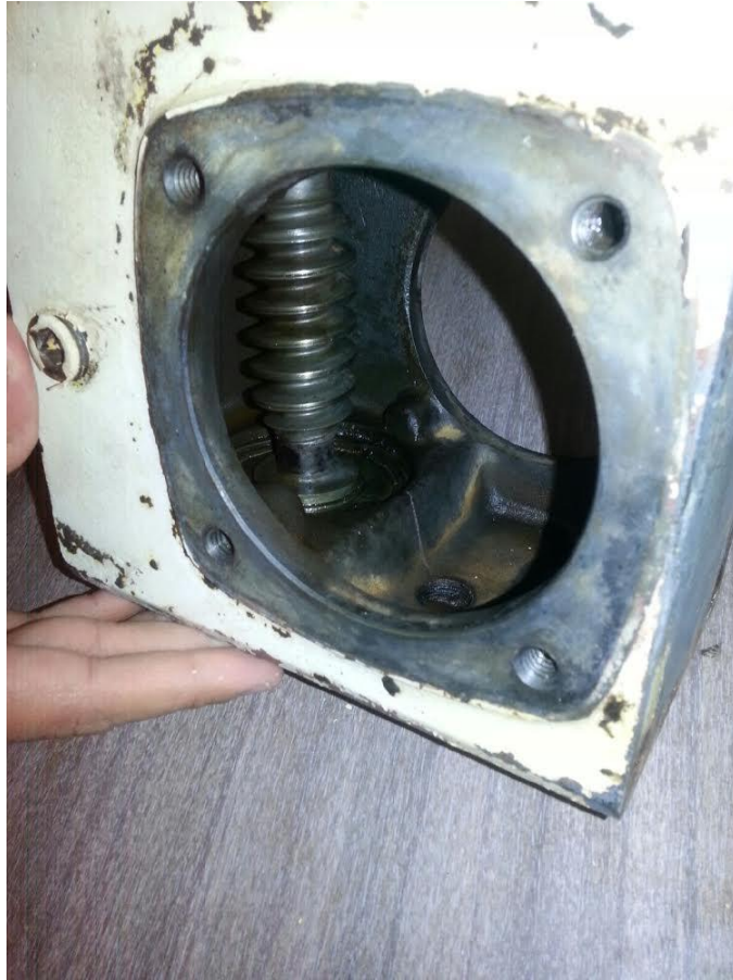
Figure 16 -Post-cleaning lower gearbox
