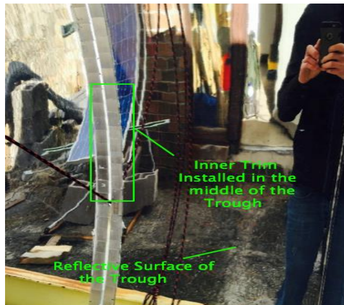
Figure 15- Inner trim installed
