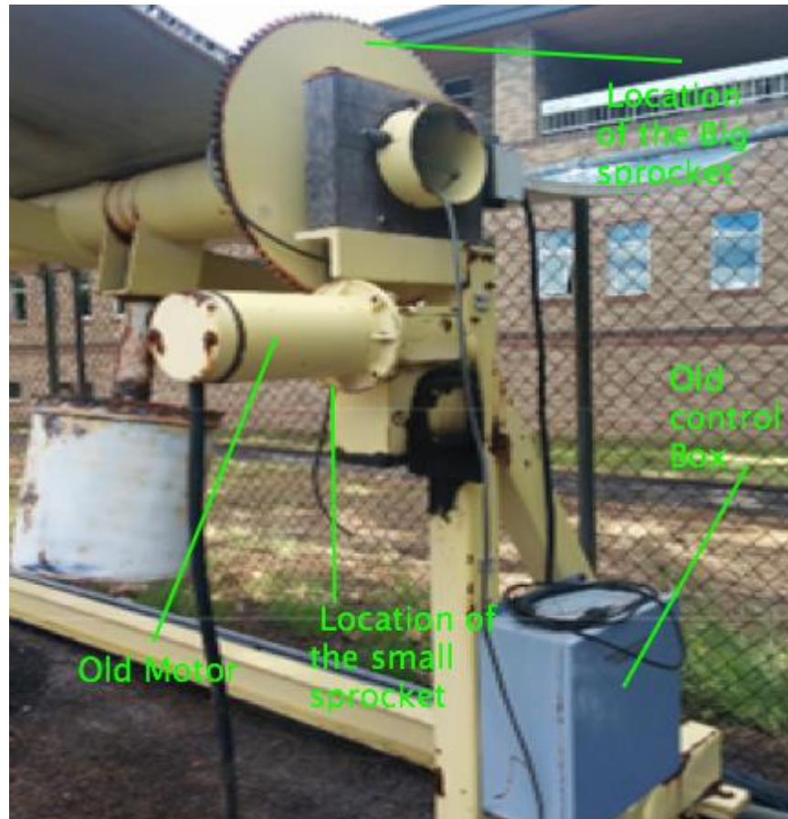
Figure 4 - Big Sprocket with missing chain
