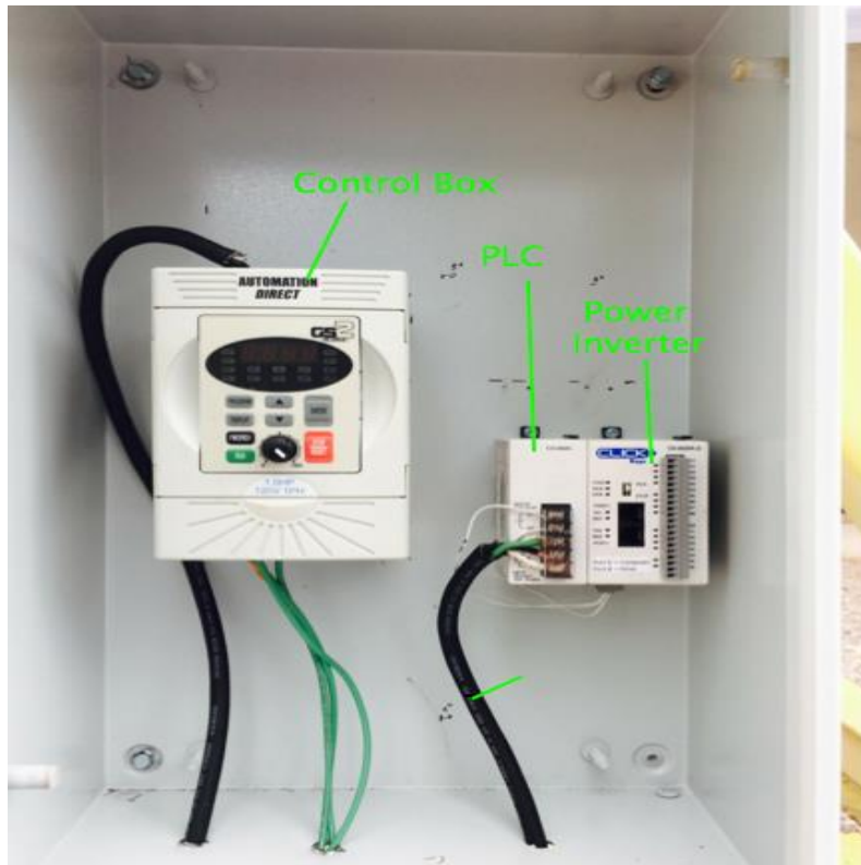
Figure 23 - Control box and components
