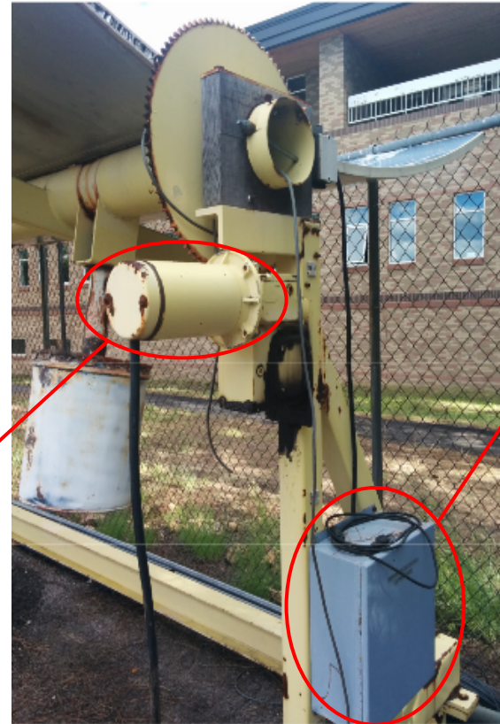
Motor and Control Box Location Picture
