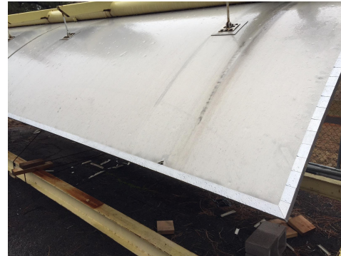
Picture4: Installed Trim
