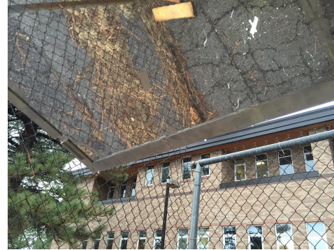
Picture3: Installed Trim
