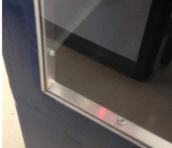
Figure 17: Window and Frame
