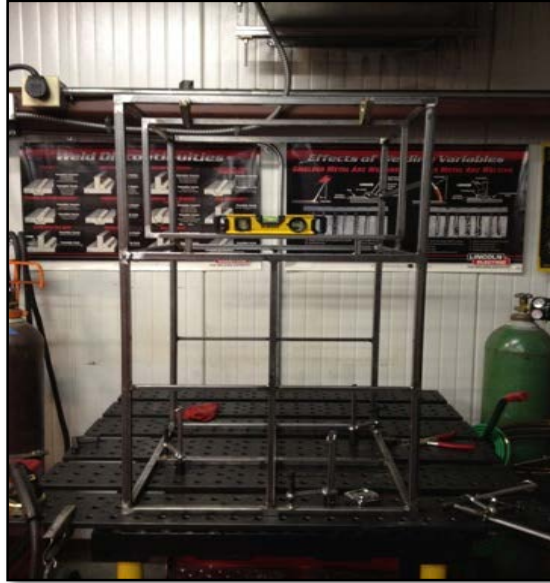
Figure 23: Frame with members welded
