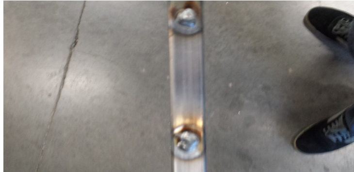
Figure 10: Welded bolts to angle support
