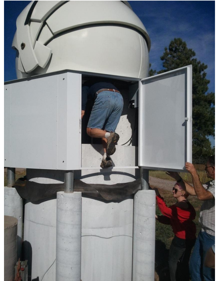
Telescope and Siderostat currently under construction
