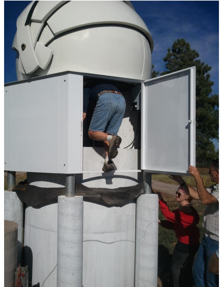
Telescope and Siderostat currently under construction
