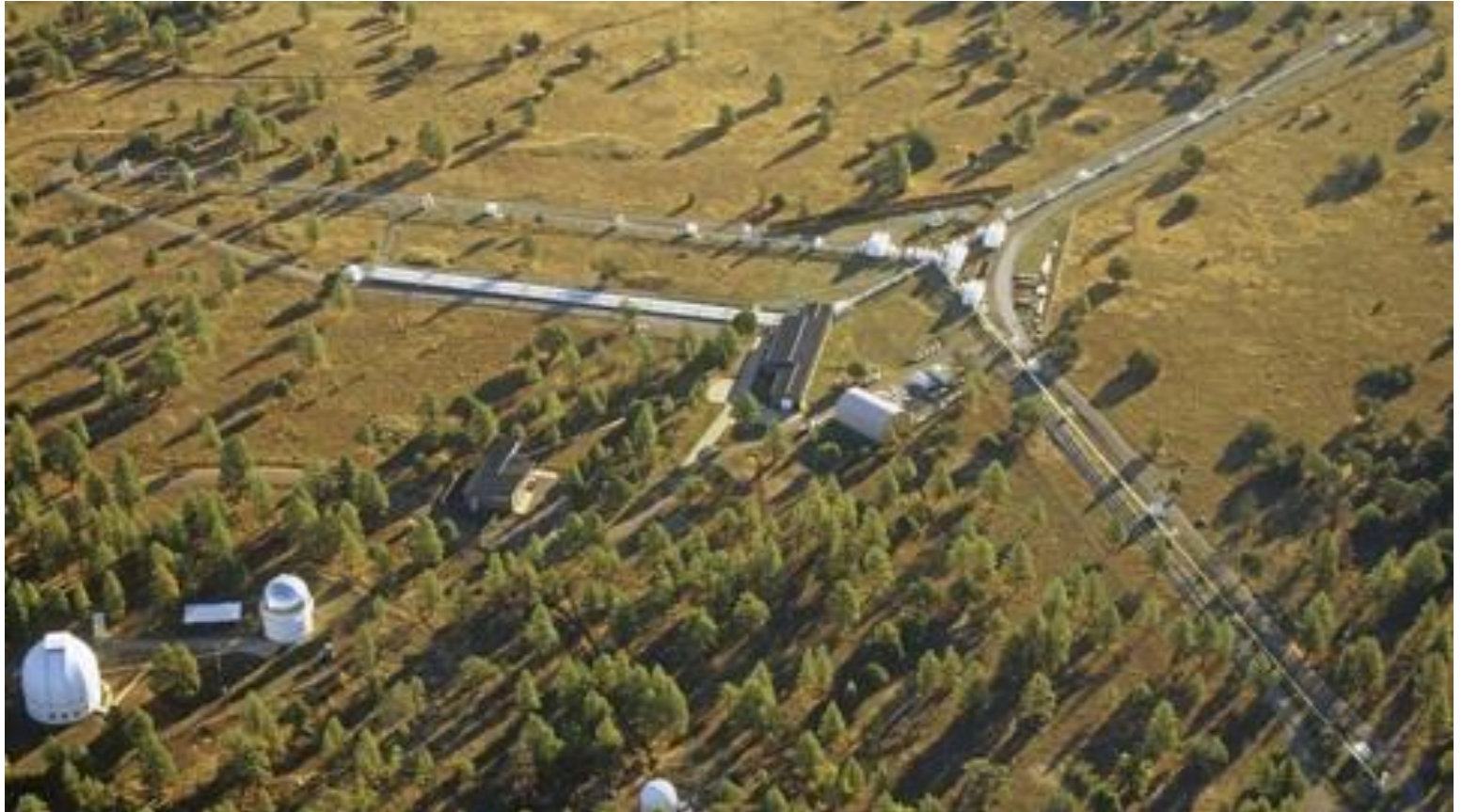
Aerial view of the NPOI facility
