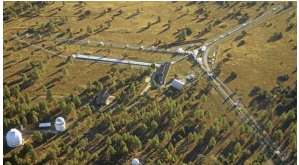
Aerial view of the NPOI facility
