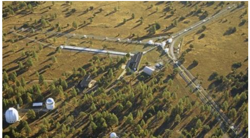
Aerial view of the NPOI facility
