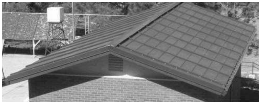
Figure 2.3.1.a. : PV cells of the Solar Shack
