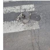
Figure 5: Pothole Patch - 1899 Bar
