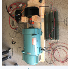
Figure 5: Generator Load Test
