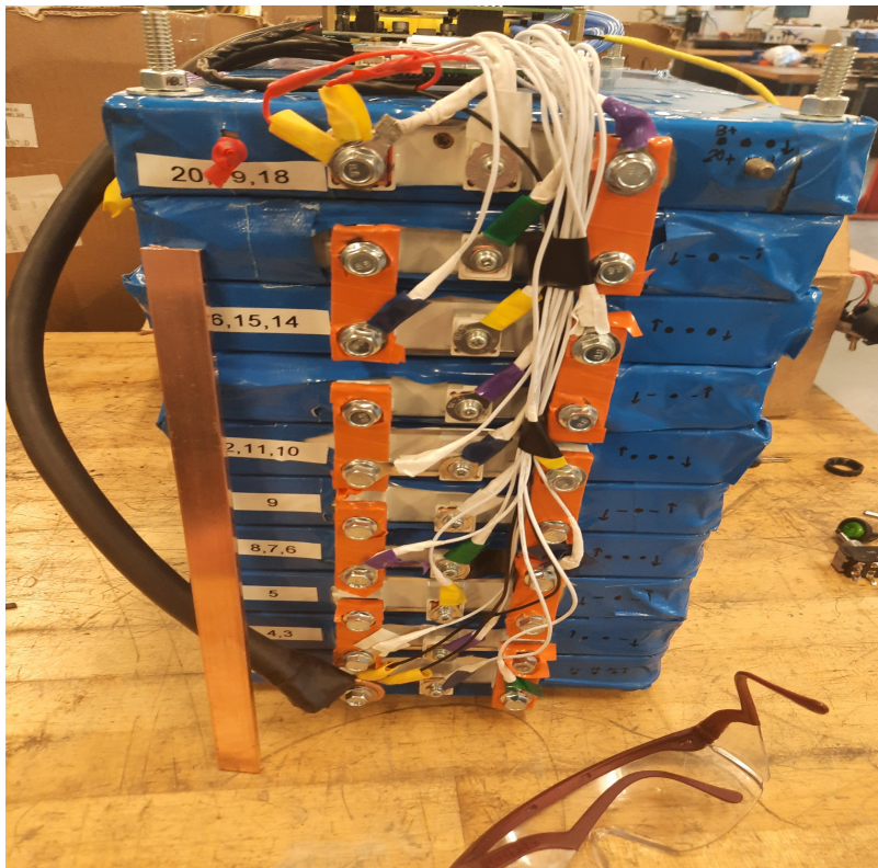
Figure 10 - BMS cell wiring
