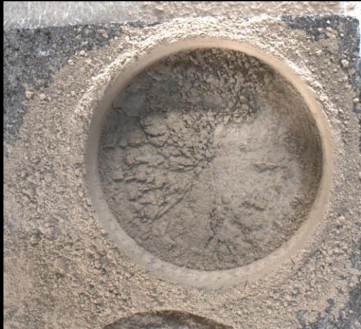
Figure 3.0. Before dust removal
