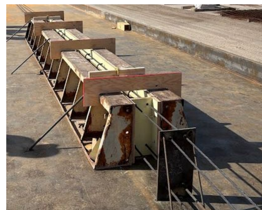
Figure 3: Big Beam Fabrication
