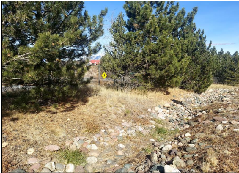
Figure 1-4: Downstream view of Existing Channel near I-17 offramp to McConnell Dr.
