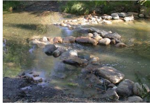
Cross-Vane Weir Channel Flow Control
