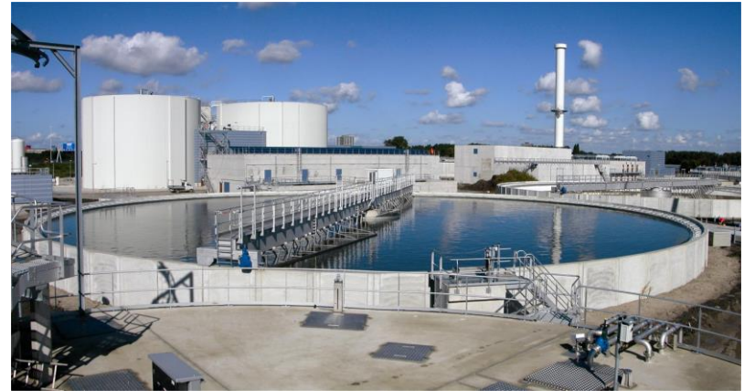
Figure 6: Wastewater Treatment Facility [5]
