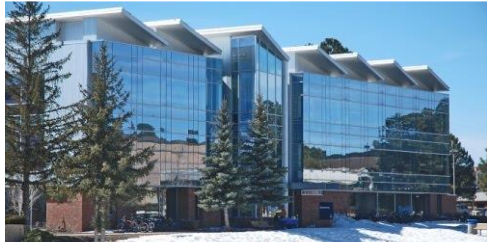
Figure 9: NAU Engineering Building [8]
