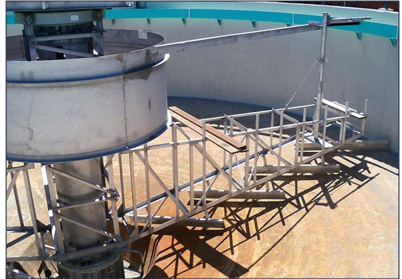
Figure 11: Column Support Clarifier Example [11]
