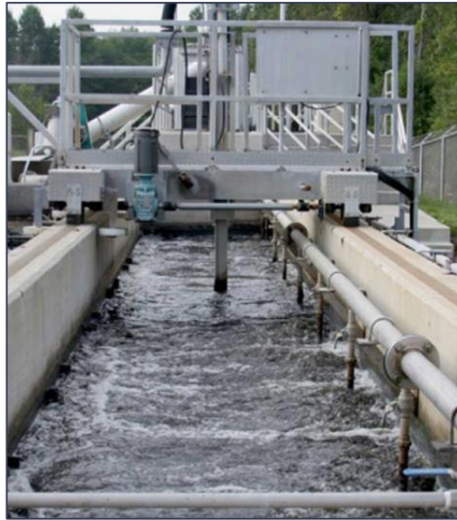
Figure 6: Horizontal Flow Grit Chamber Example [7]
