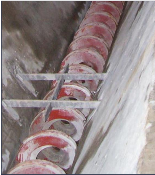
Figure 5: Aerated Grit Chamber Example [6]
