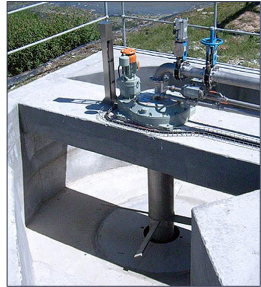
Figure 7: Vortex Grit Chamber Example [8]
