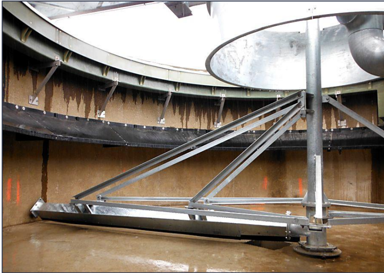
Figure 10: Bridge Support Clarifier Example [10]
