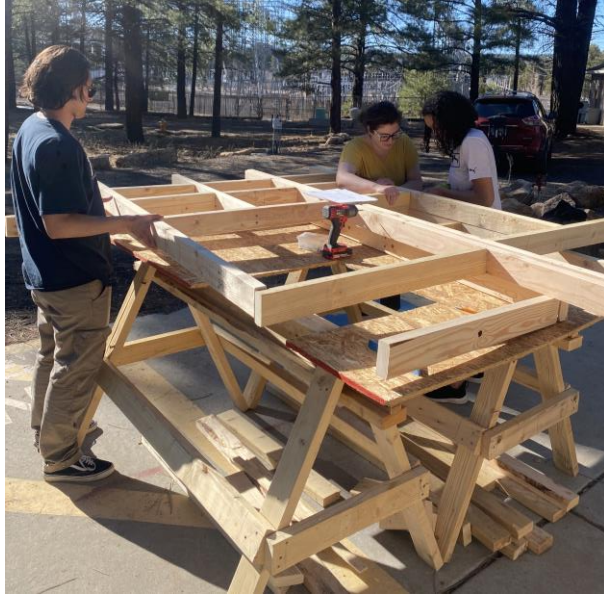
Figure 6- 2: Floor Diaphragm
