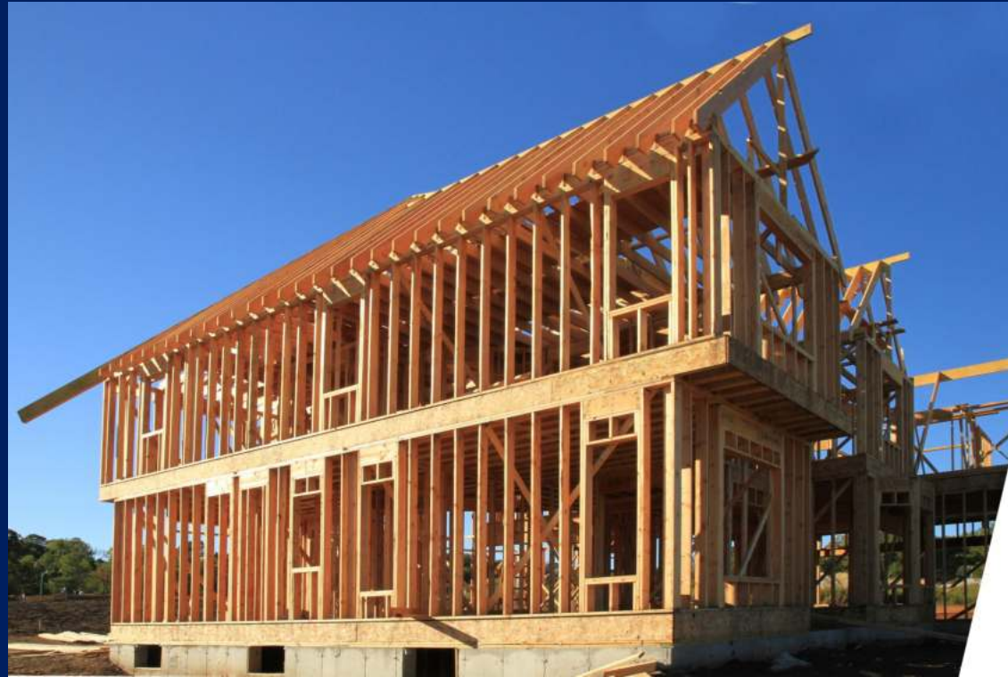
Figure 24: Timber House Framing [10]
