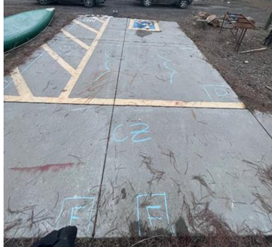
Figure 6-2 Construction Site CEMCEE FIELD Station
