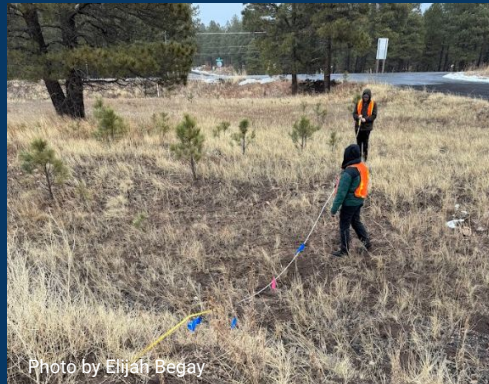
Figure 30: Surveying the typical cross section
