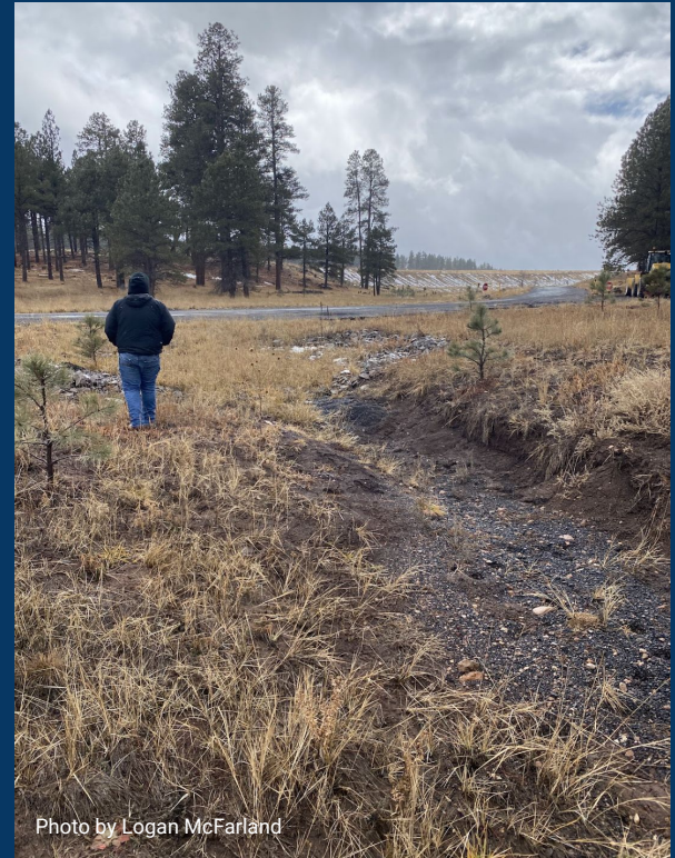
Figure 34: Looking upstream of existing channel
