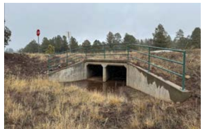
Culvert at the furthest point downstream of channel
