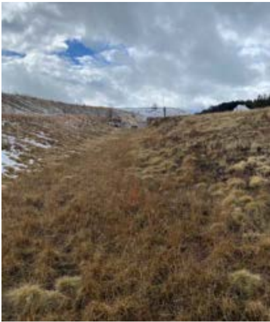
Existing shallow concentrated flow channel
