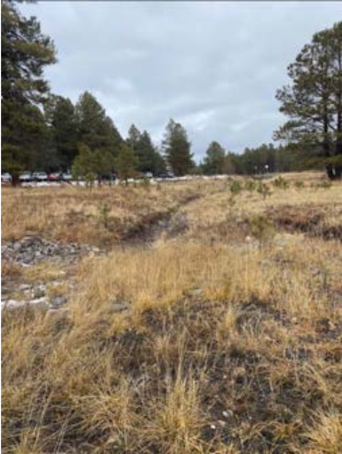
STA 0+00 looking downstream of the existing channel
