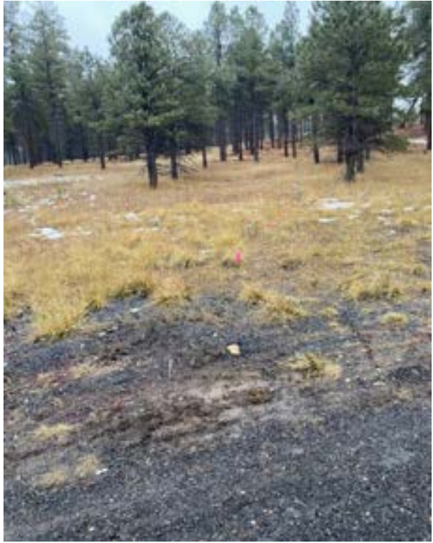
Staking out the upstream side of the channel
