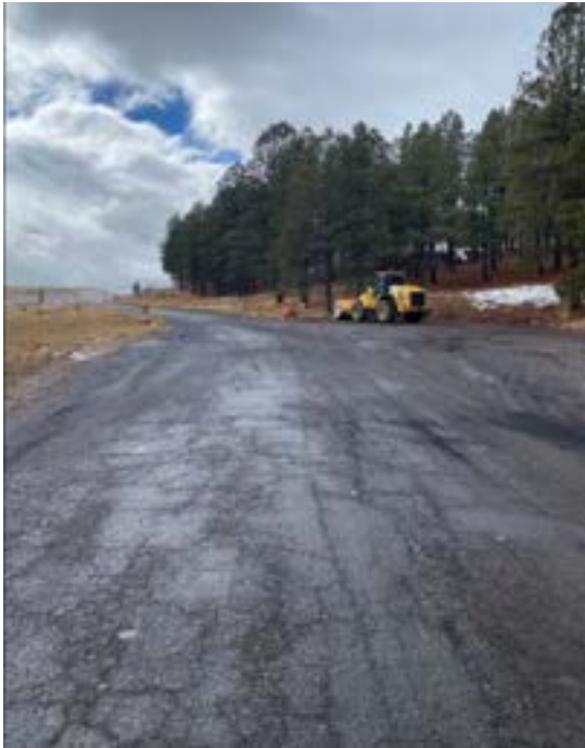
Graded road from the east side of site
