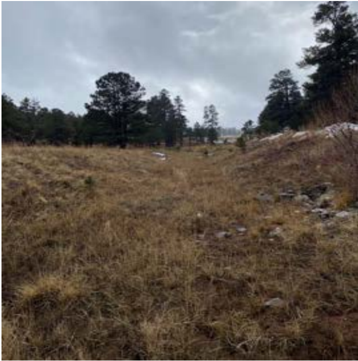
Existing channel (looking upstream)
