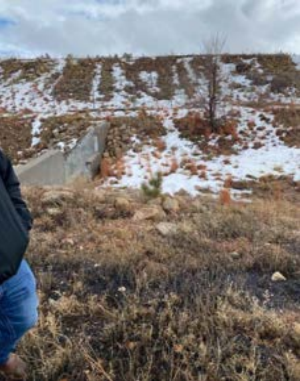
Upstream side of the Weir
