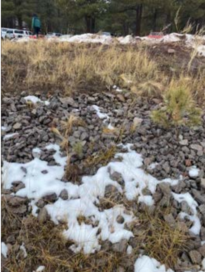
Riprap at the furthest upstream point of the existing channel
