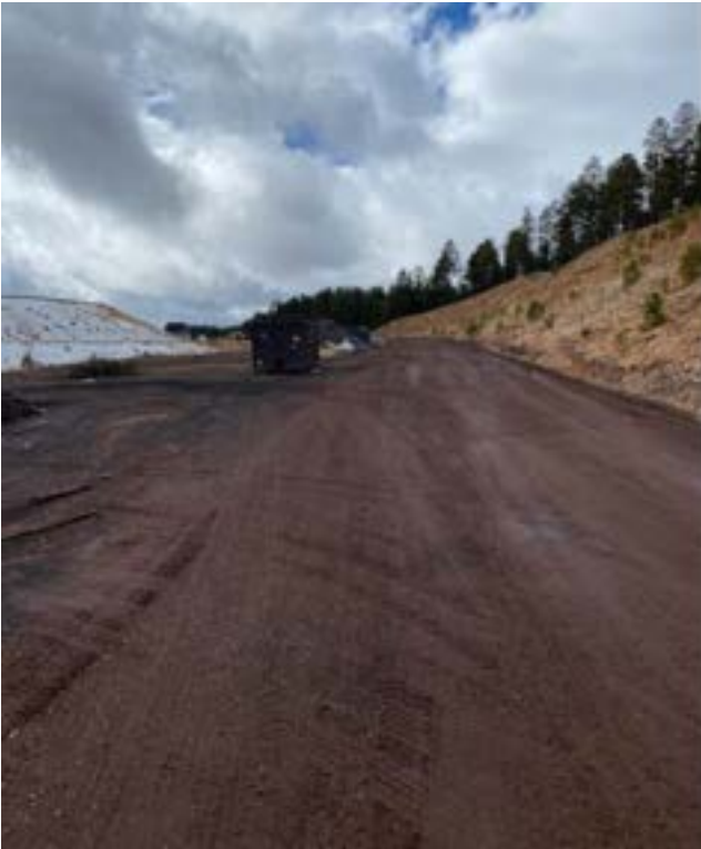
Midpoint of the proposed roadway
