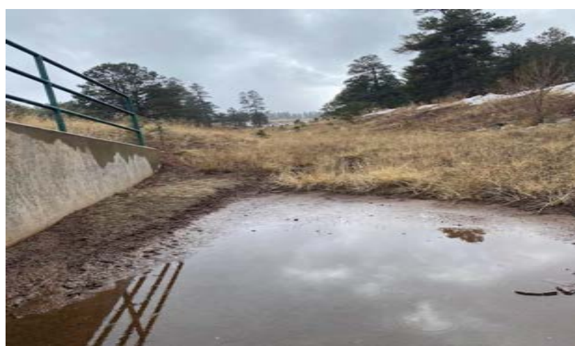
Looking upstream of the channel
