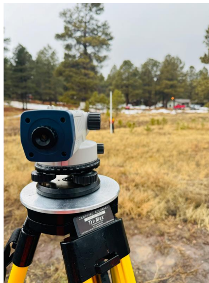
Figure 3-1: Surveying existing channel
