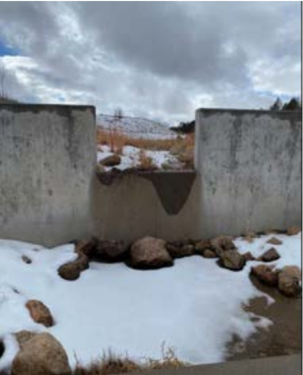
Closer view of the weir
