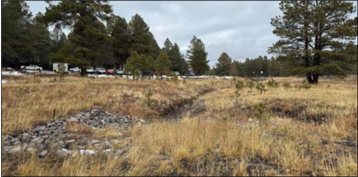
Figure 3-5: Looking downstream of existing channel
