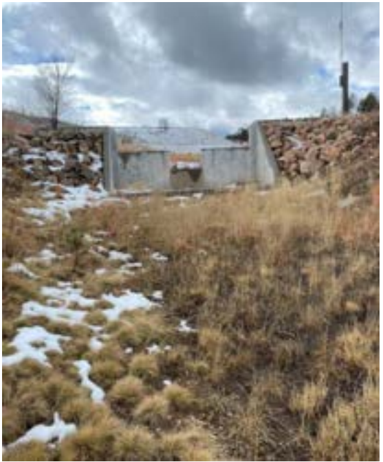
Existing weir further upstream
