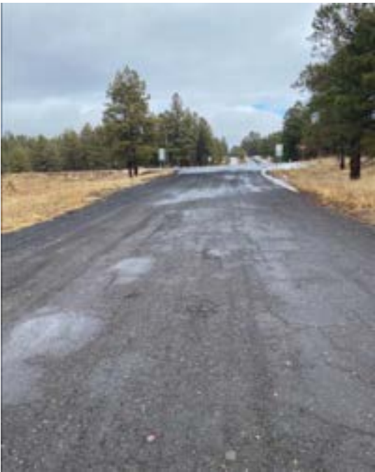
Graded road from east side of site
