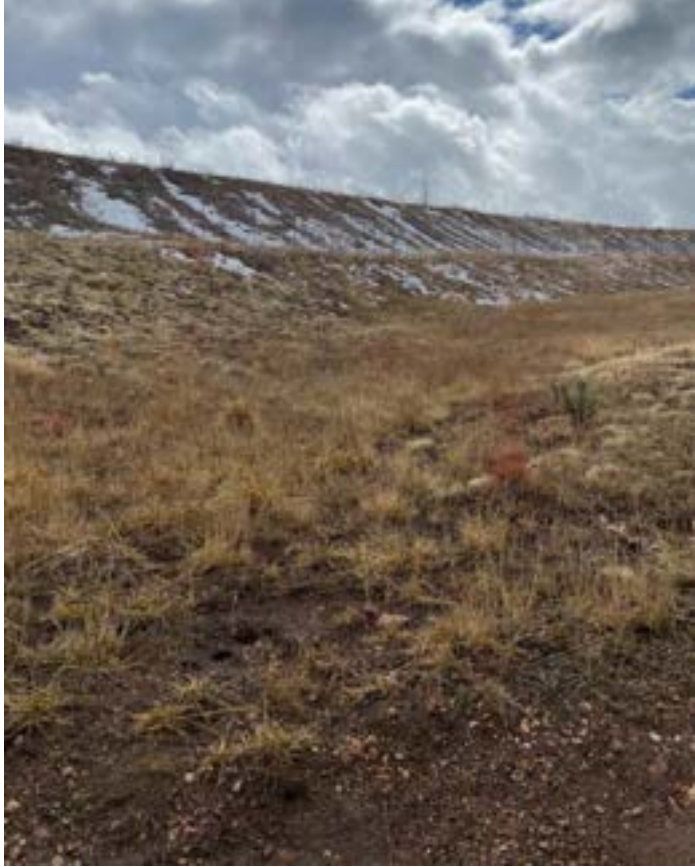
Existing wash with airport security fence along the upper ridge
