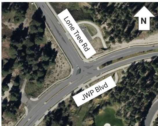
Figure 15, JWP Blvd & Lone Tree Rd Intersection
