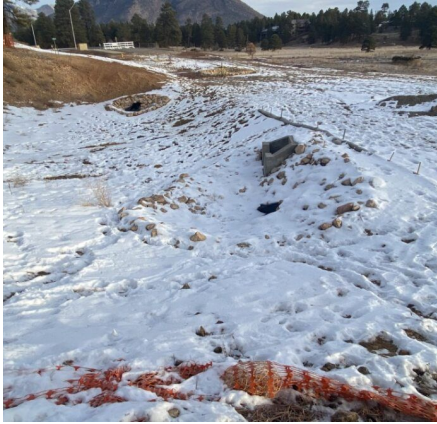
Figure 2, East Terminus Culverts Credit: James H
