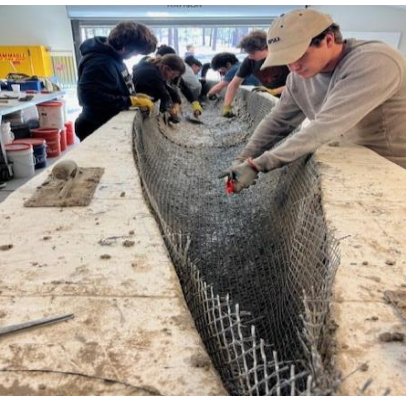
Figure 5: Primary Reinforcement Placement
