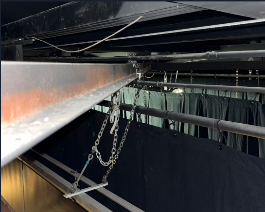
Figure 11: L 3"x2"x1/4" Cross Brace [1]
