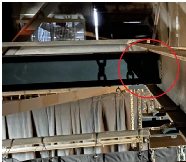
Figure 22: Photo Verification of Beam to Beam Connection
