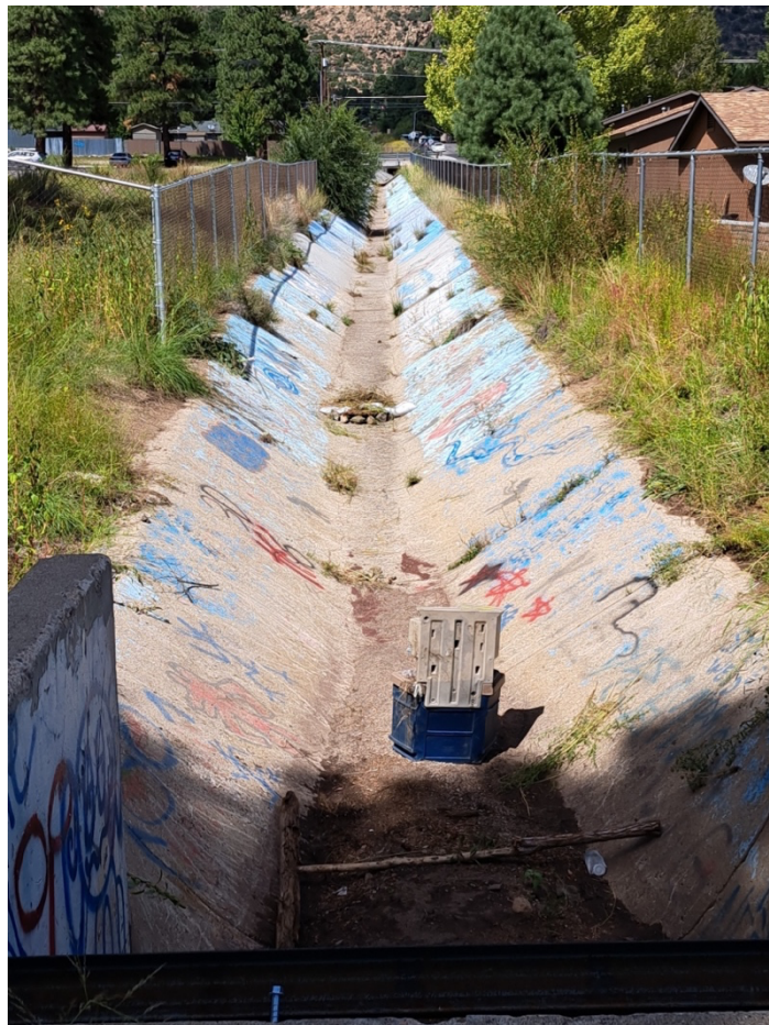
Figure 1-4: Existing Channel at E, Elder Dr (Siler Homes)
