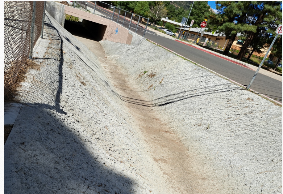
Fig 7: Culvert and open channel in project site Credit: Sneha Joshi
