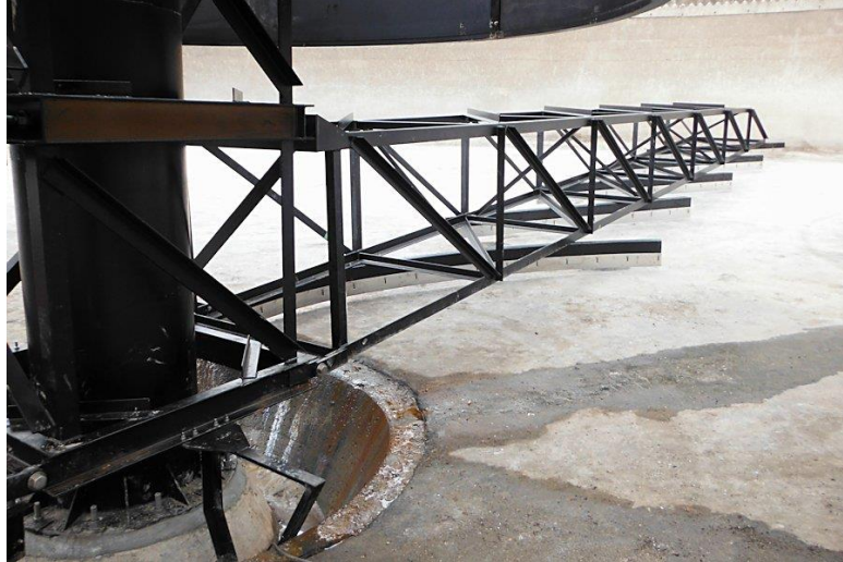
Figure 5. 10 Column Support Clarifier [32]
