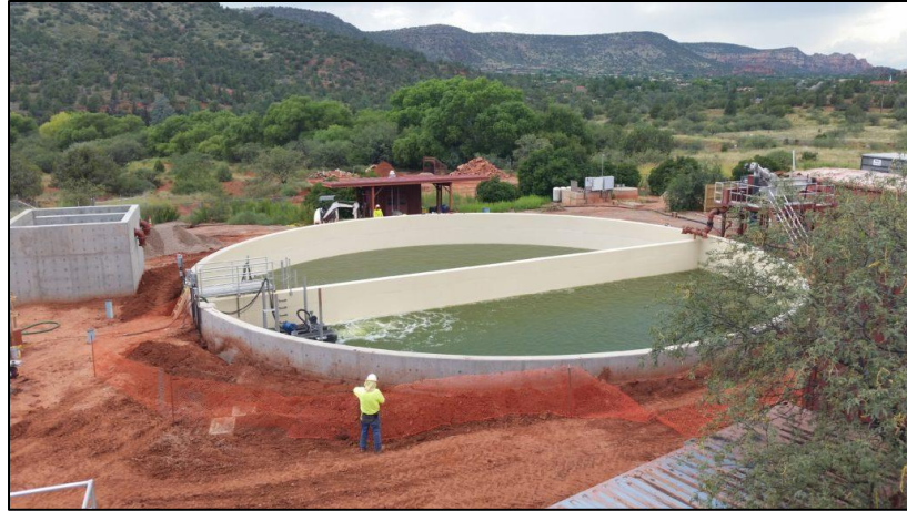
Figure 5. 8 In-line Equalization Basin [30]
