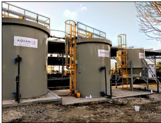
Figure 5. 15 UASB Reactor [38]
