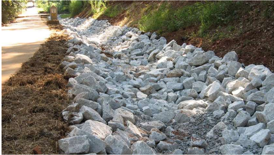
Figure 5-4 Typical Erosion Protection [10]
