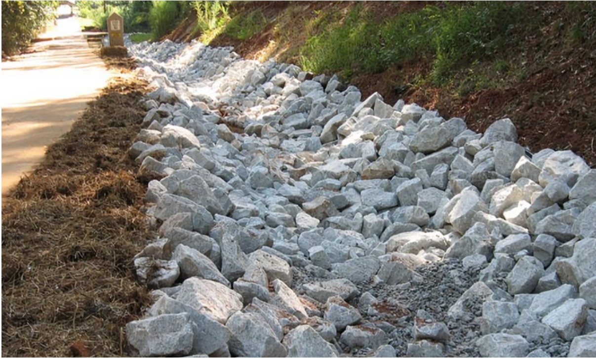
Figure 9 Typical Erosion Protection [1]
