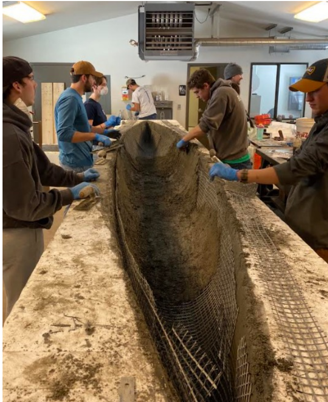
Figure 15: Placing Reinforcement Picture Credit: Hunter Kassens
